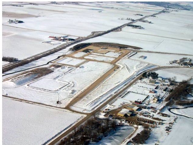
Dyersville Ethanol under construction
