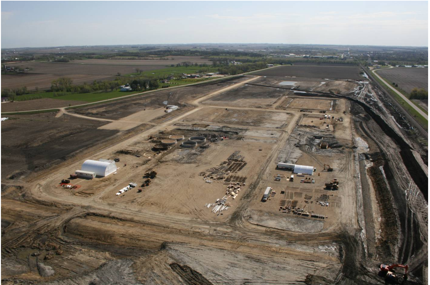
Photo of the new Ethanol plant on April 29, 2007
