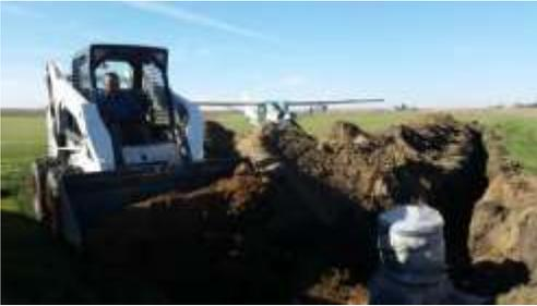
Fred Lansing backfills the septic and lays the drain field.
