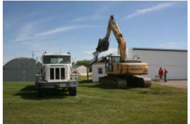
Lansing Brothers Construction remove old lounge
