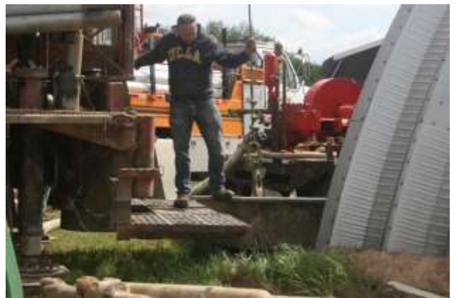
The well gets dug
