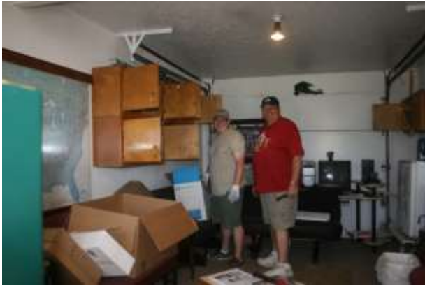
Ron and Nick Radloff empty old lounge for destruction
