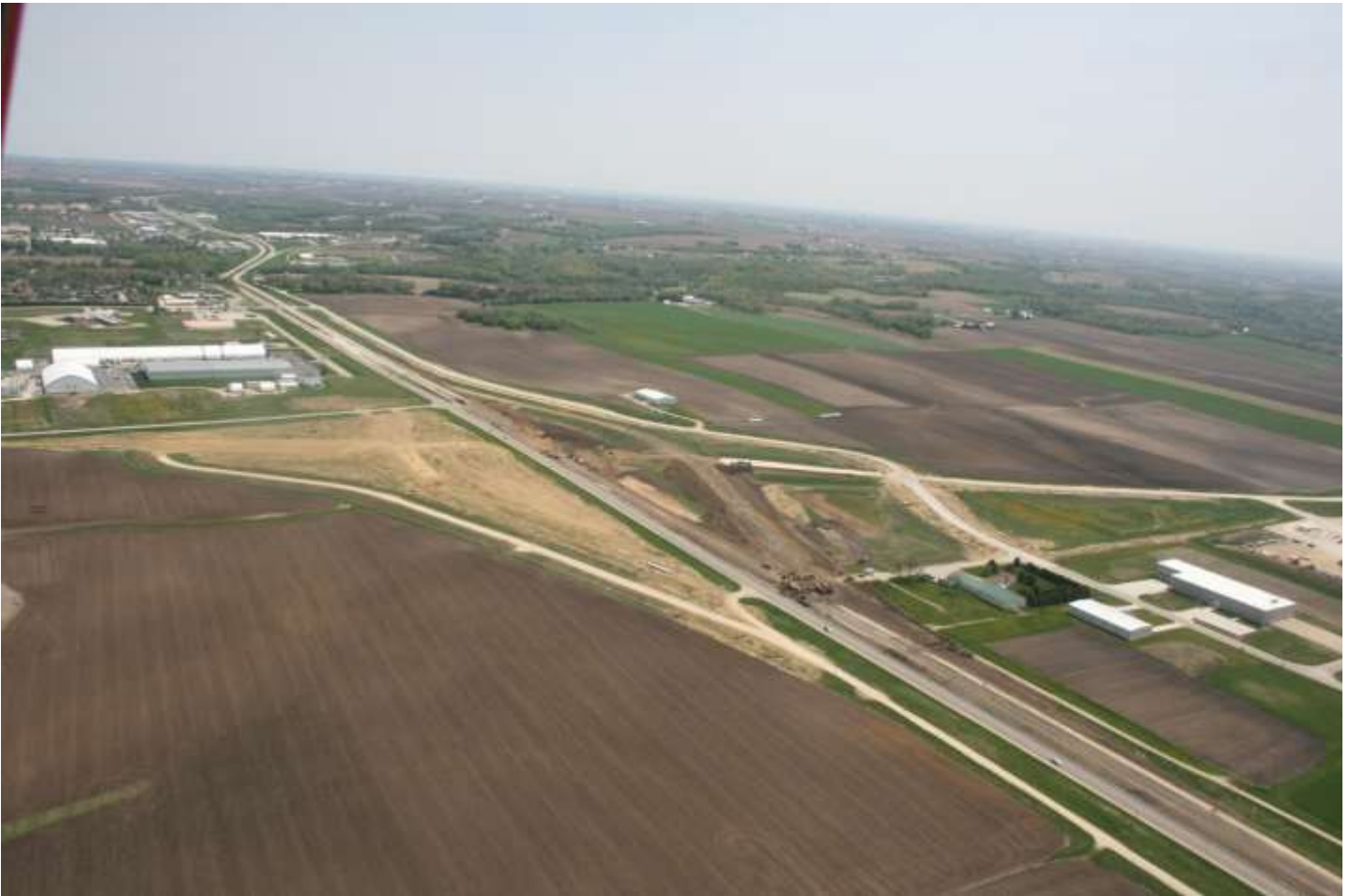
Hwy 20 interchange construction continues.
